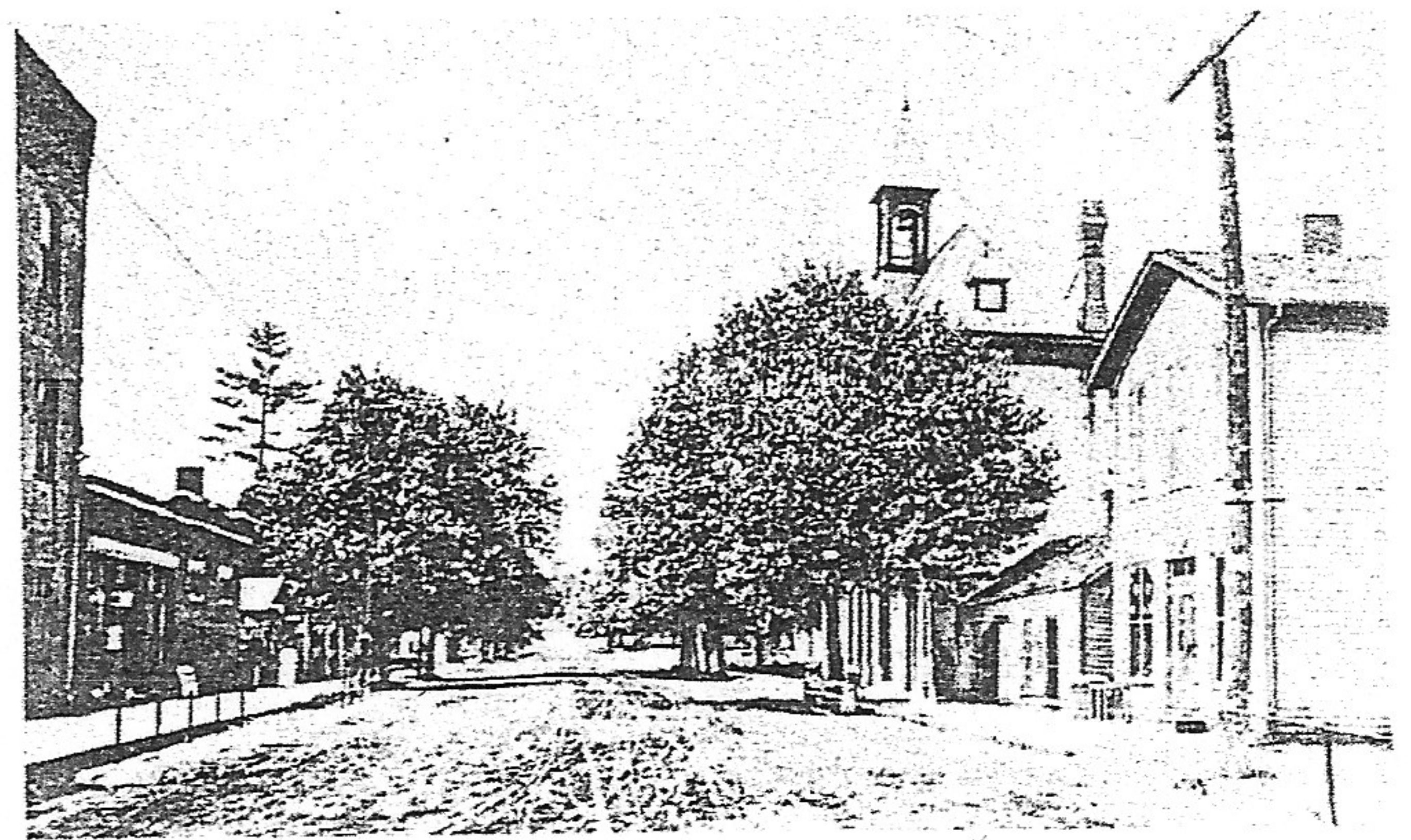
West Central Ave. — 1920
