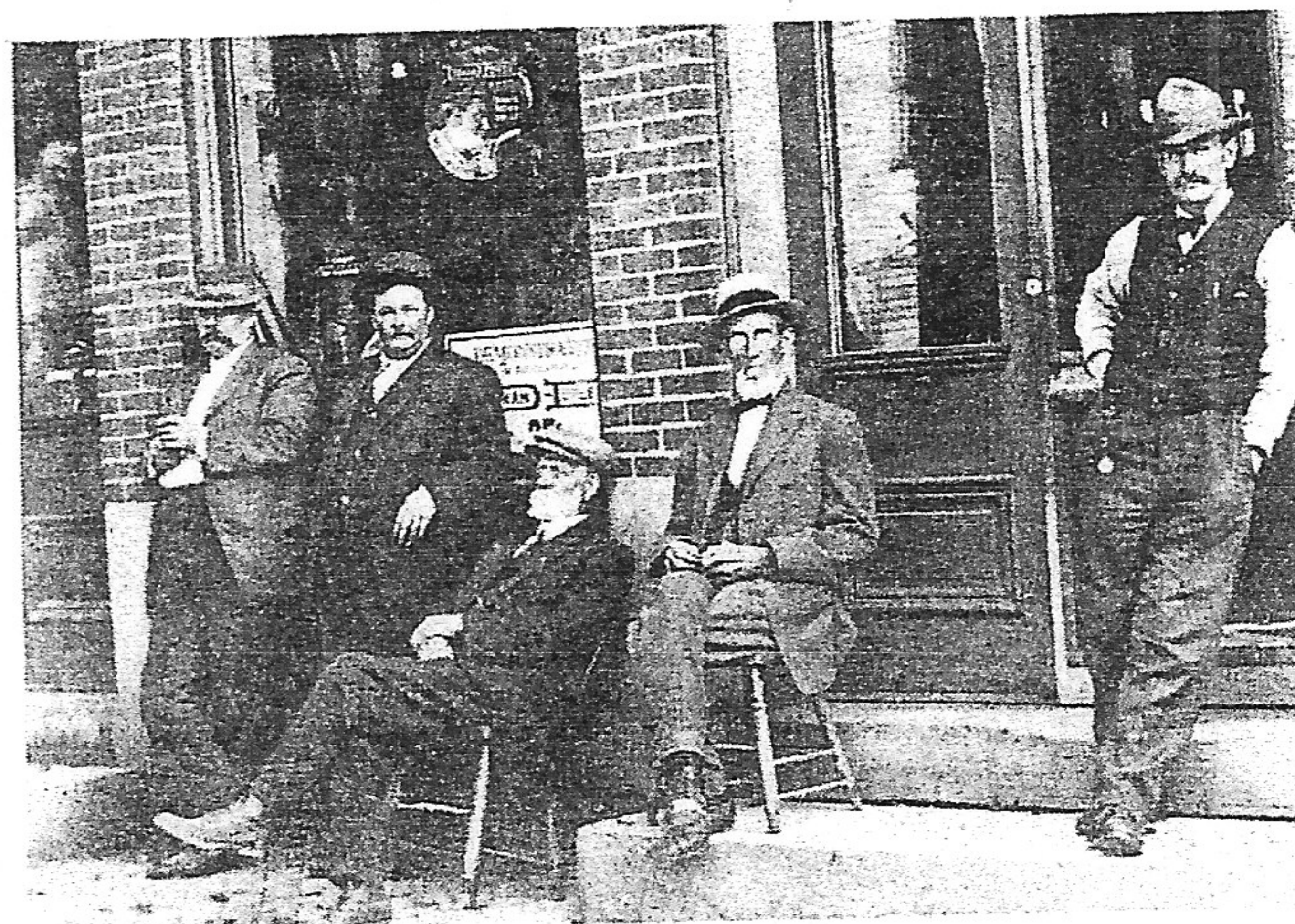
McCord's Hardware Store about 1900. Now Caskey's Display Room
